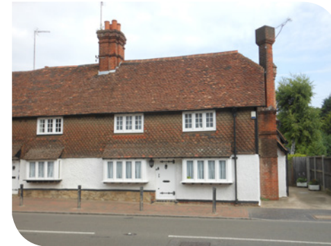
Clay tile roof and tile-hanging
