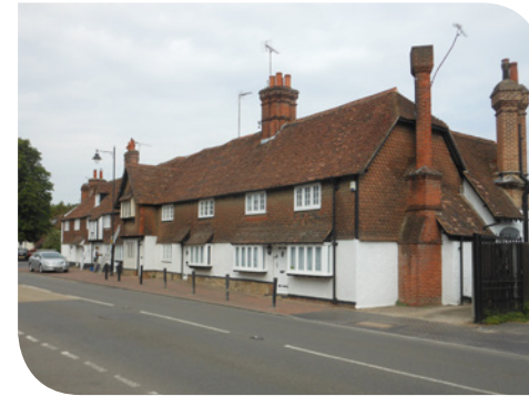
Tall brick chimneys
