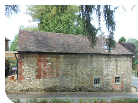
Rubble stone walls
