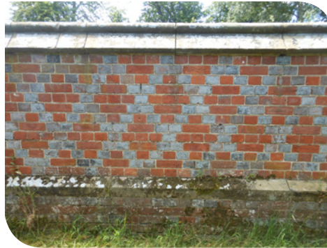
Brick estate wall to Hall Place
