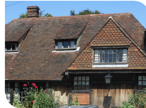
Clay tile roofs and tile-hanging
