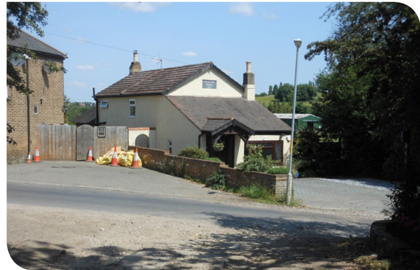
Lack of front boundaries detracts from the character of the conservation area
