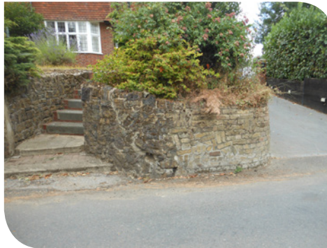
Stone and brick retaining wall
