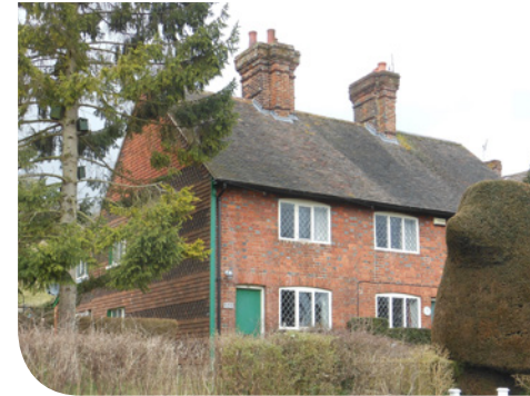
Unbroken roof slopes
