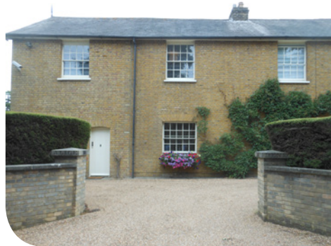
Yellow brick and slate roofs
