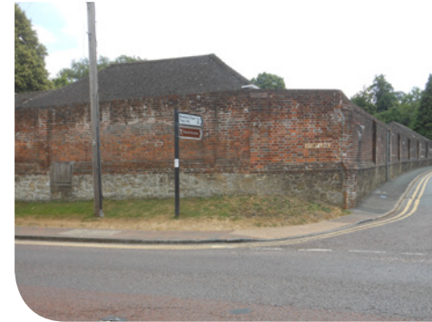
Kentish ragstone and brick walls
