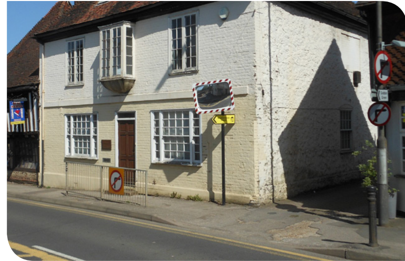
Traffic and other signage harming the setting of listed buildings on the High Street
