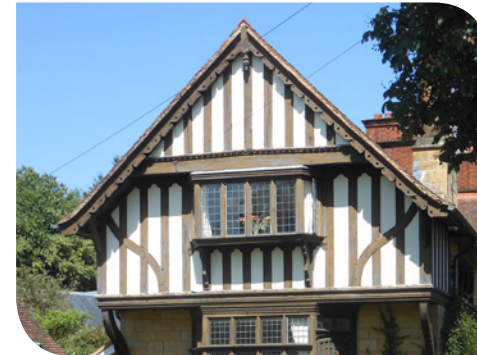
Steeply pitched roofs
