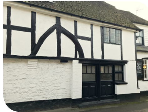
Rubble stone and timber frame
