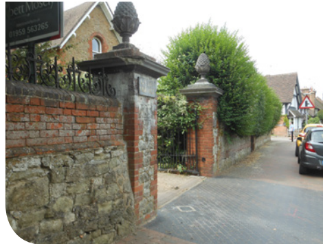
Substantial gate piers
