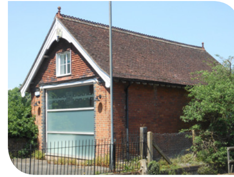
Clay tile roofs with decorative ridges
