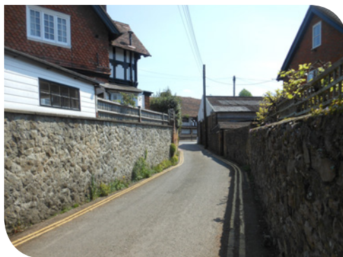
Kentish Ragstone walls
