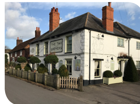
Tall brick chimneys
