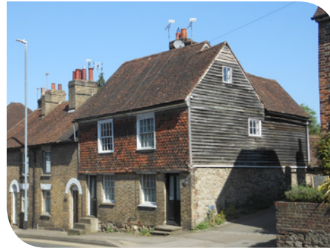
Tile-hanging and weatherboarding
