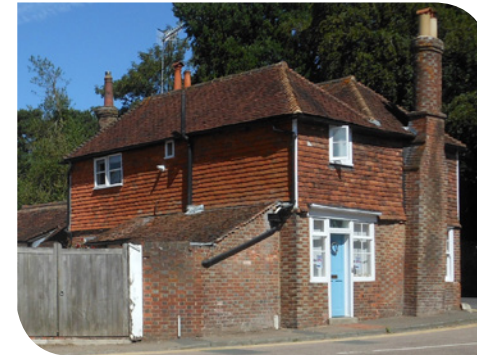
Clay tile roofs and tile-hanging
