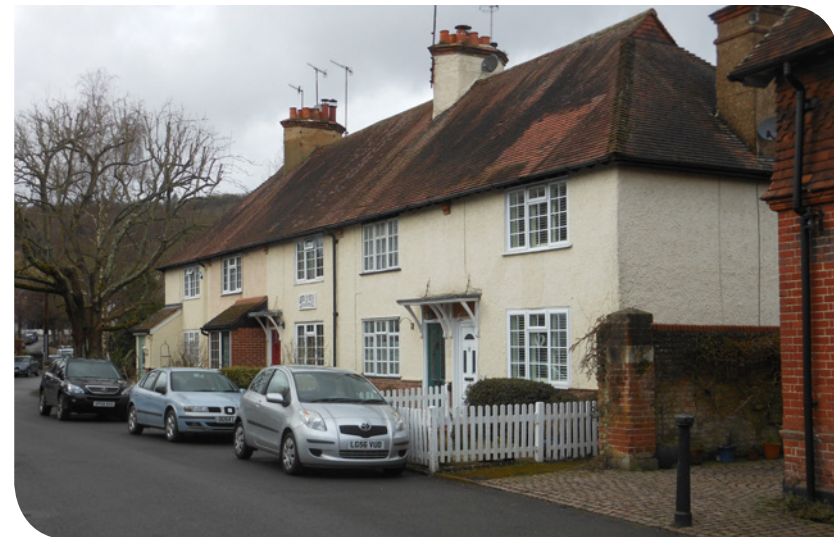
Loss of unity of a terrace of houses due to later additions
