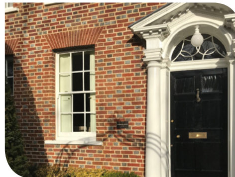
Flemish bond brickwork
