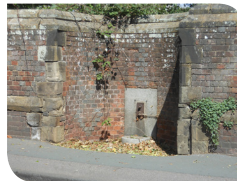
Drinking fountain in the park wall
